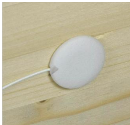
Fit the cap, making sure the outlet is in the desired position (do not jam the cable). Glue the cap if necessary.
